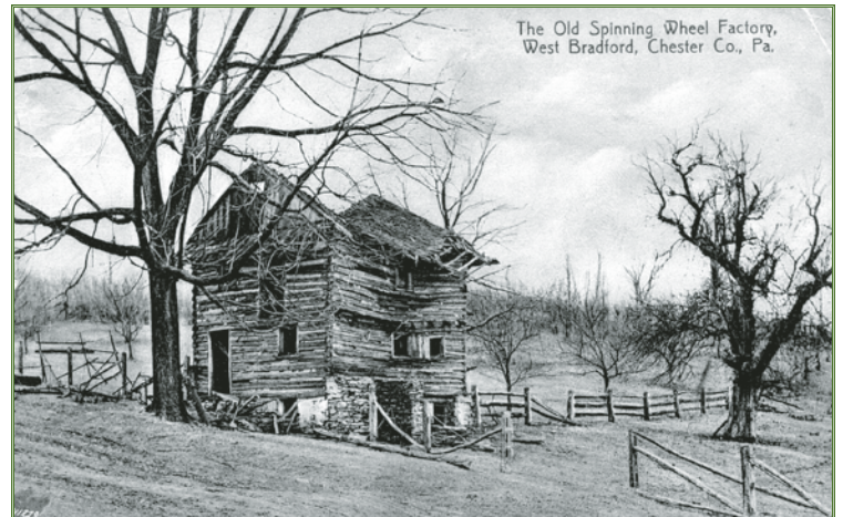
Above: Sugar's "spinning wheel factory" was located just north of Sugar's Bridge crossing the East Branch of the Brandywine. Part of the foundation could still be seen during the 1940's.
